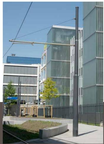
The use of trams or trolley buses is the future: it is a proven form of sustainable public transport without annoying exhaust fumes in the urban environment. Especially for this purpose we have already been able to provide many tram and trolley bus routes with poles for suspending the necessary overhead contact lines. Thanks to the overhead contact lines the passing tram or trolley bus is provided with power in a reliable manner.
